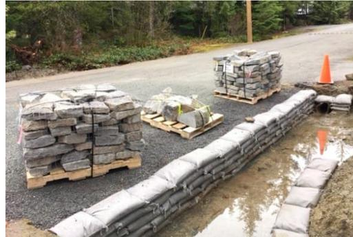
The dry-mixed concrete in the bags reacts slowly with moisture from pre-wetting and environmental exposure to form a hardened concrete installation. The bags will slowly weather away, leaving an attractive "pillow block" structure.
